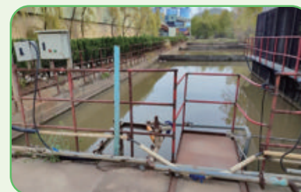
A rainwater and sewage sedimentation tank is arranged next to the raw material incoming road, and is used for flushing the raw material warehouse road
