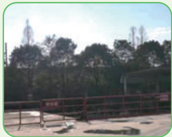
Rainwater collection pond
