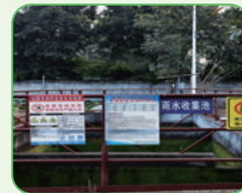
Rainwater collection pond
