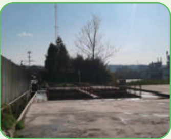
Truck washing sedimentation tank
