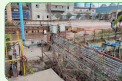
A sewage sedimentation tank is arranged next to the truck wheel washing machine at the side door of the shipment, and th
