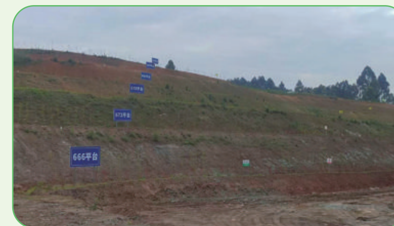
Completion of temporary slope planting on the north side of the mining area by the Tazishan Mine
