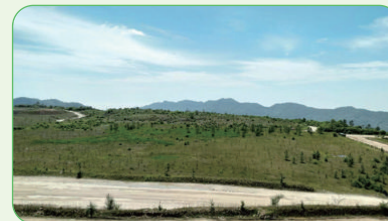
Completion of temporary slope on the north side of the mining area by the Tazishan Mine
